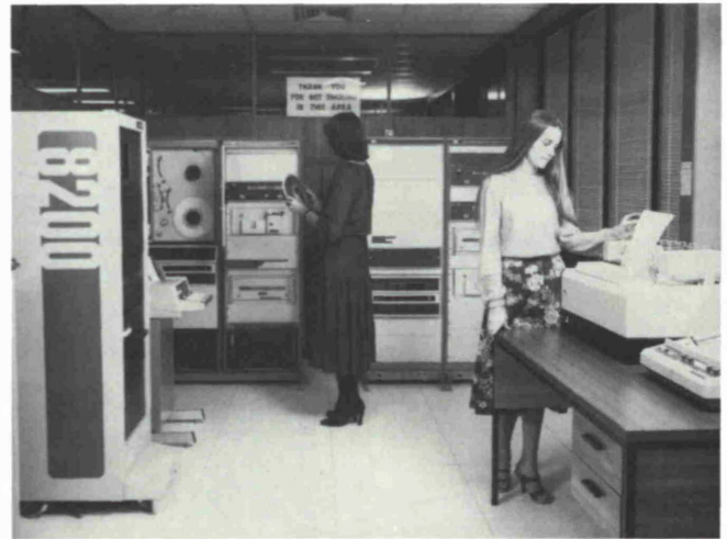
Fig. 12: Computer centre showing plant monitoring and commercial computer
