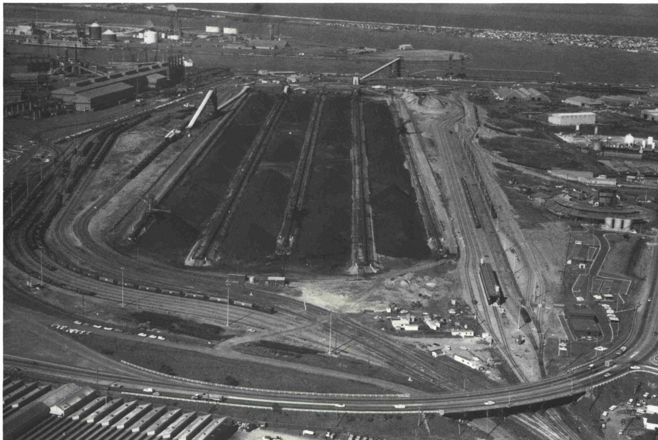
Fig. 2: PWCS coal handling facility at Port Waratah, 1978
