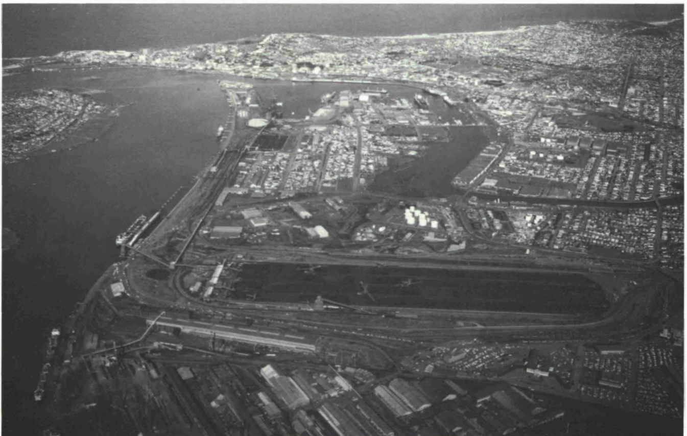
Fig. 4: Port of Newcastle showing coal export facilities
