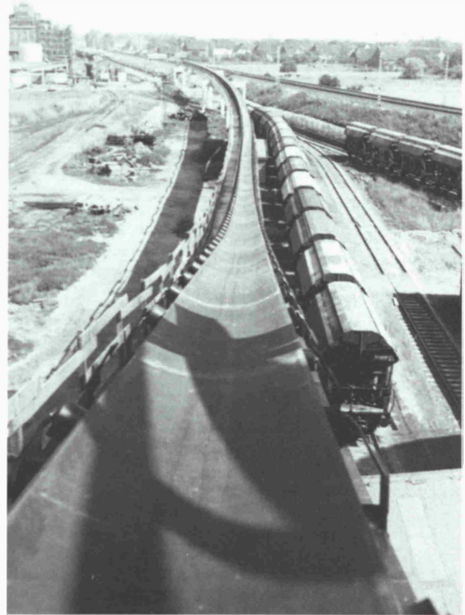
Fig. 3: Belt conveyor system for potassium salt
