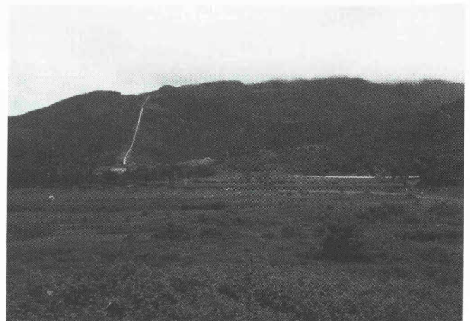
Fig. 11: View of the steeply descending portion of the conveyor shown in Fig. 10 together with the first horizontal curve
