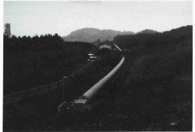
Fig. 7: Belt conveyor system for lime-stone
