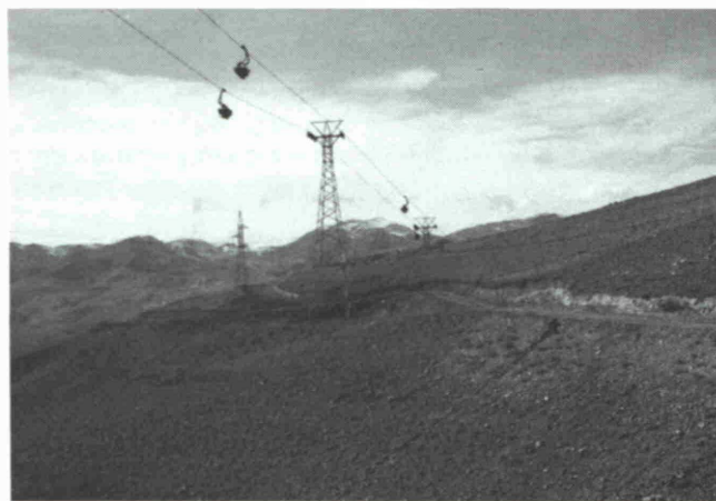
Fig. 1: Ore-carrying monocabable aerial ropeway crossing over a barren stretch of country in the edge of the Khamseh mountains in Iran
