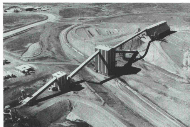
Fig. 7: Aerial view of coal storage facility at Clovis Mine in Wyoming
