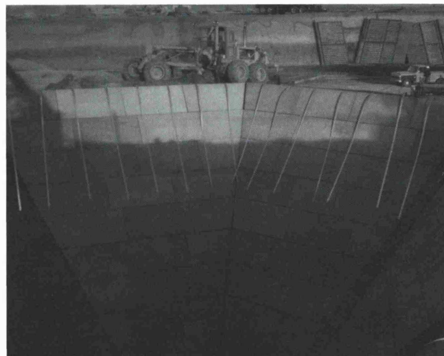
Fig. 6: Endwall construction for the 100,000 t storage barn at Black Thunder Mine
