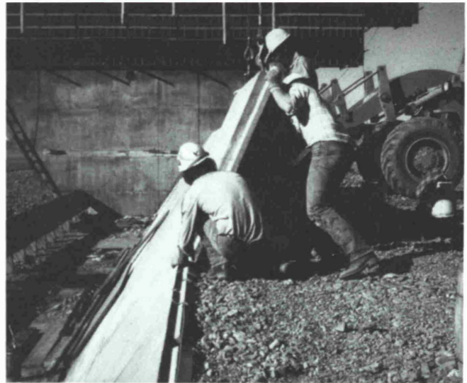
Fig. 3: Positioning of a panel in the early stages of construction
