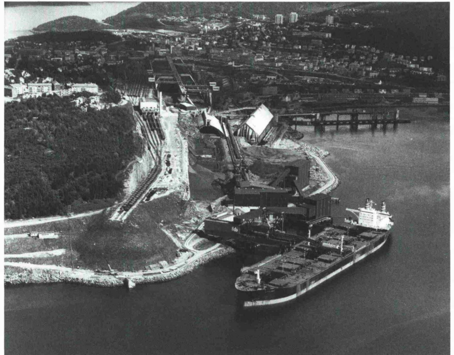
Fig. 2: Narvik: Last expansion stage — new berth stockyard and screening plant. Railway yard, unloading station. Old stockyards and pier in the background. Loading of the largest vessel so far — 280,000 dwt.
