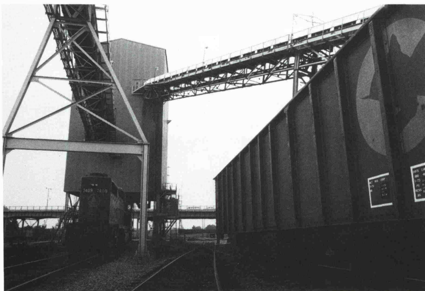
Fig. 2: View of the rail loadout
