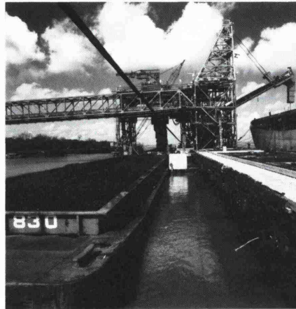
Fig. 4: Resurfaced original dock provides good access between new dolphins
