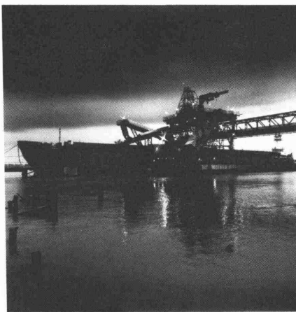
Fig. 8: A 13,000 ton capacity gulf barge moored at the new Plaquemines Parish Terminal will deliver Illinois coal to powerplants on Florida's west coast
