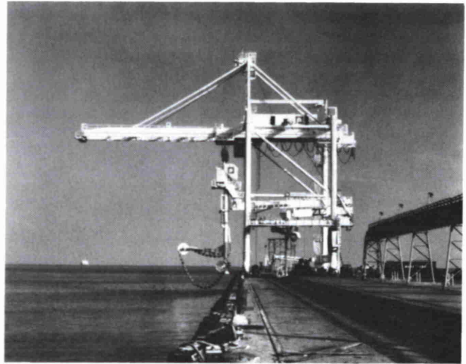
Fig. 8: Side view of Gulfport installation showing the bucket line, digging arm and dockside take-away conveyor
