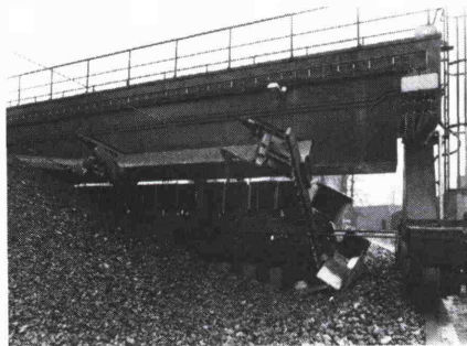
Fig. 2: View showing the carrying cells for the careful handling of coal
