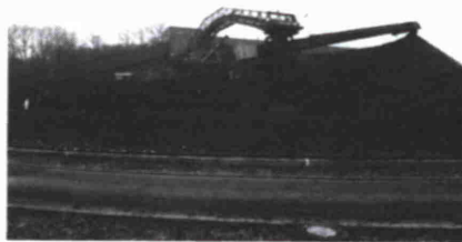
Fig. 1: General view of the circular stockpile system: Gewerkschaft Sophia Jacoba , Hückelhoven, Germany
