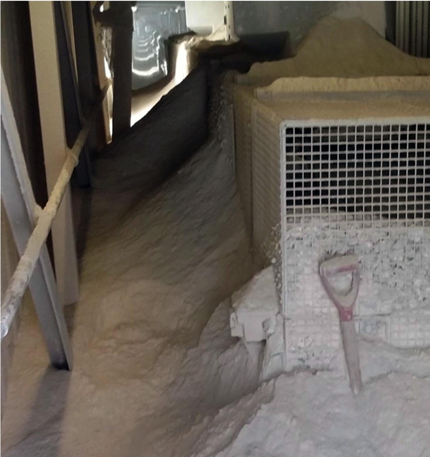
Piled high enough to encapsulate the tail pulley, the dust blocked walkways, posing a potential hazard.
