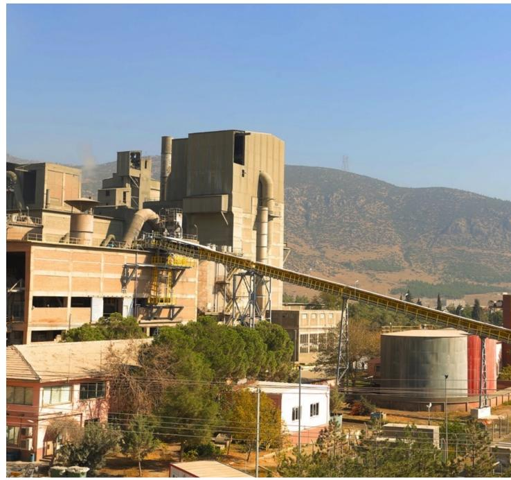
The conveying system is eco-friendly, requires low maintenance and its enclosed type of construction protects the environment safely from possible material falling down and emissions.
