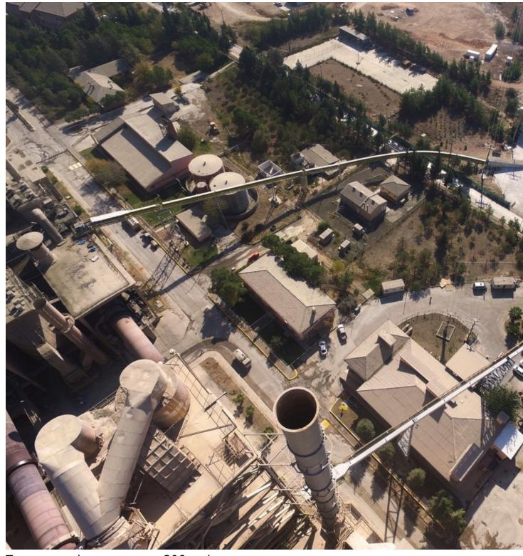
Two successive conveyors, 206 and 190 metres long, are used. Each Pipe Conveyor reaches a capacity of 15 tonnes per hour.
