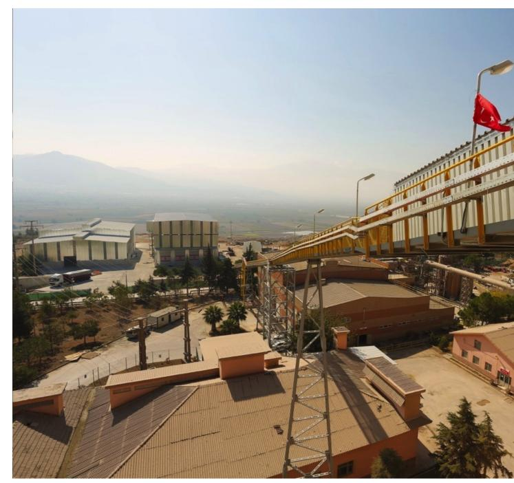
The Pipe Conveyor transports the alternative fuels from the storehouse to the preheater.
