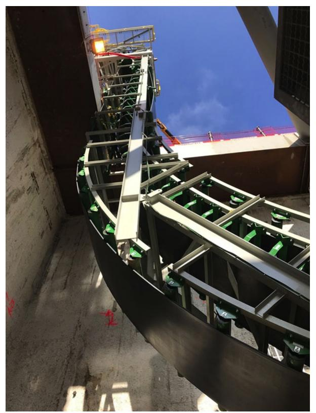
DSI GPS is able to elevate material economically, at high volumetric rates in limited vault space.
