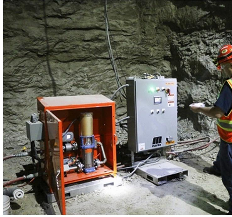
Monitors, valves and boosters are in accessible cabinets, so the system is easy to inspect and maintain.
