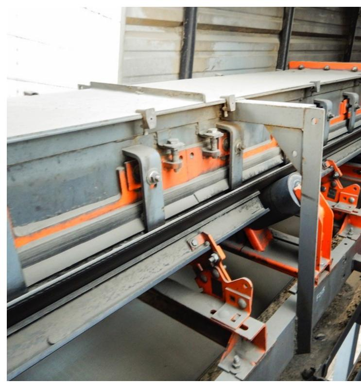
The project included upgraded transfer points to eliminate belt sag and improve sealing, as well as belt cleaning and alignment systems.
