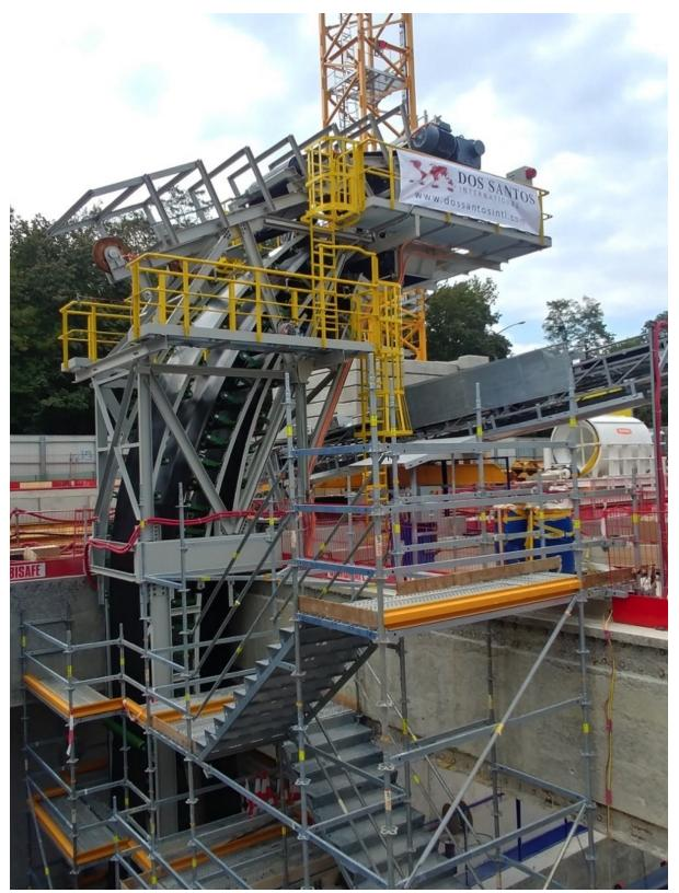
The DSI Sandwich belt high angle conveyor will elevate 800 t/h of tunnel muck at a 90° angle.
