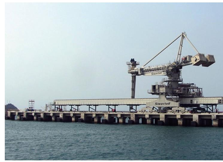
The Siwertell System at Cilegon, Indonesia includes one ST790 D-type shipunloader and two belt conveyors.
