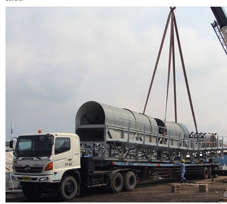
With the help of an assisting crane, the pre-assembly phase of the installation, involving the assembly of the 18 m prefabricated module sections, was completed in the space of only two days.
