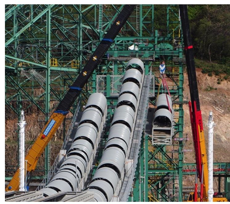
Siwertell's Modular Belt Conveyor System comprises precisionengineered, lightweight, prefabricated frame modules, which can be designed horizontally, or to various inclines.
