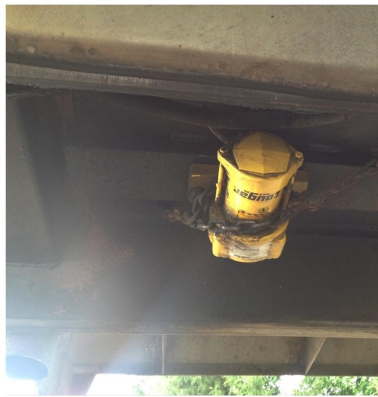
The unit is mounted to the frame and secured by a safety chain.
