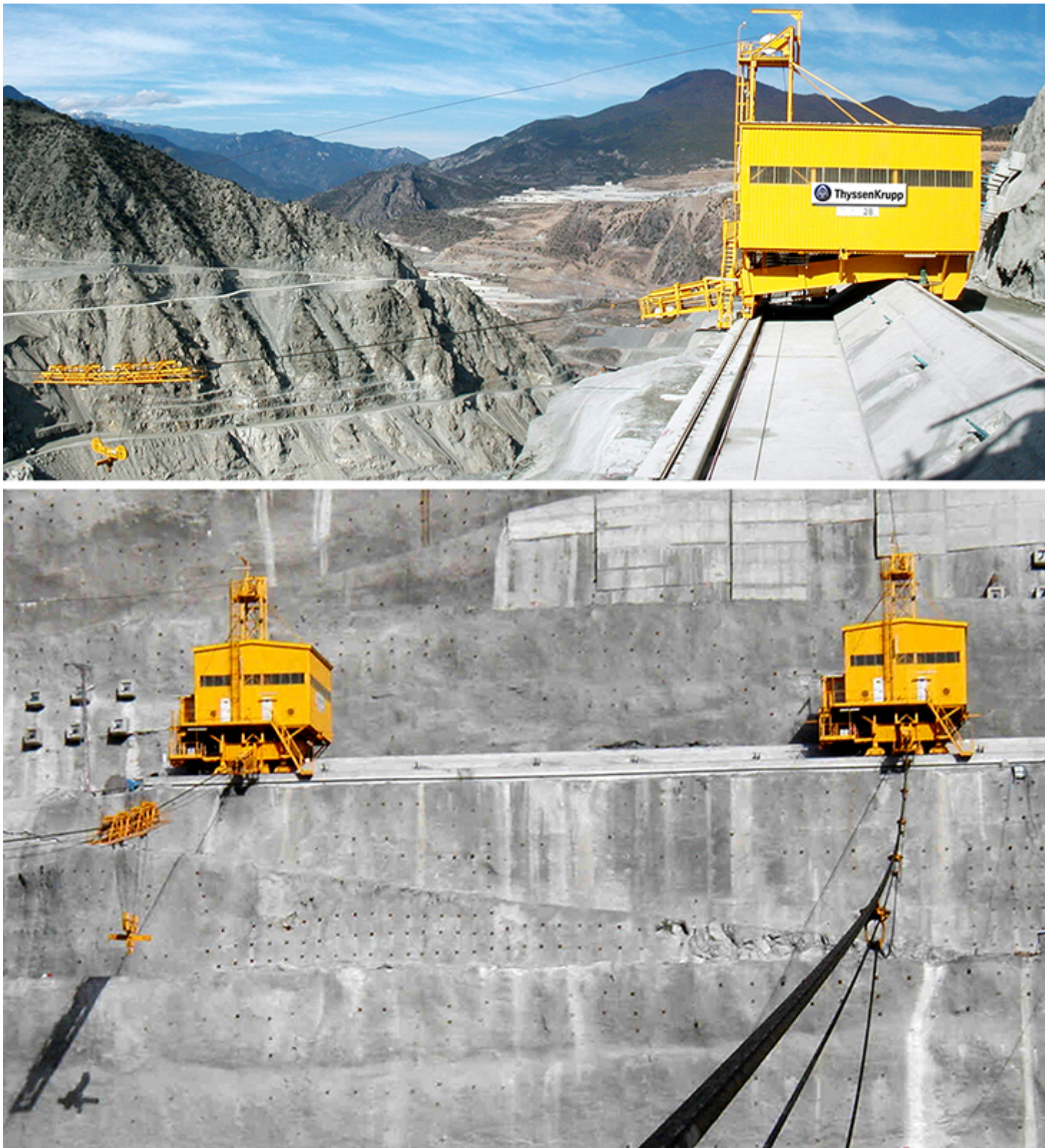
Fig. 2: Thyssenkrupp cable cranes for dam construction.
