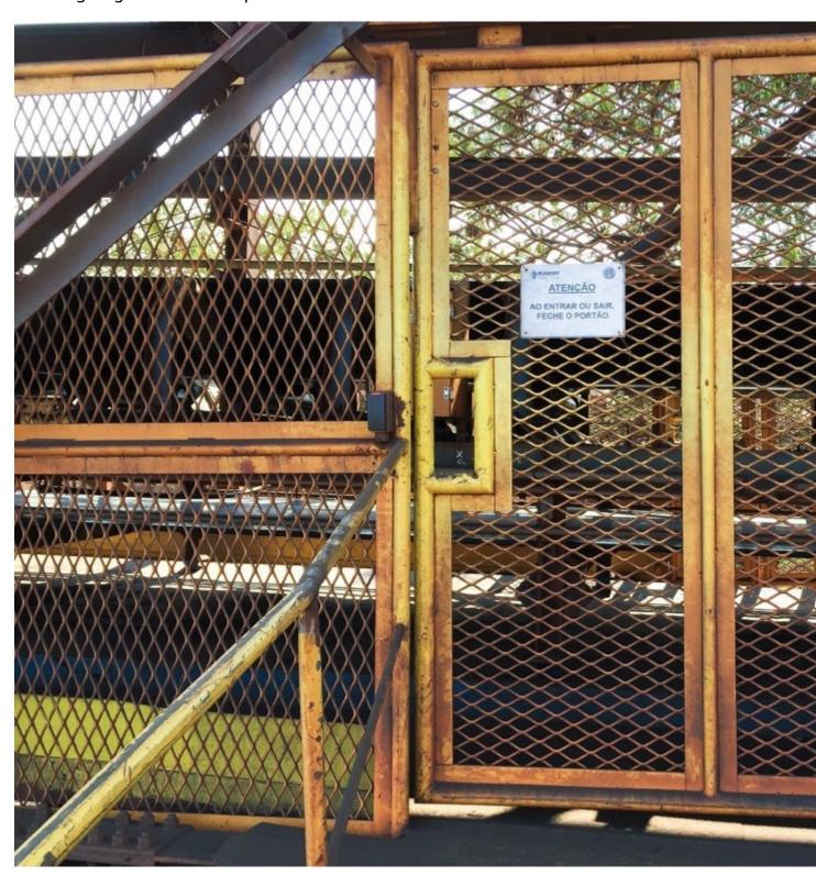
A gate to a conveyor walkway, controlled with an RFID sensor.
