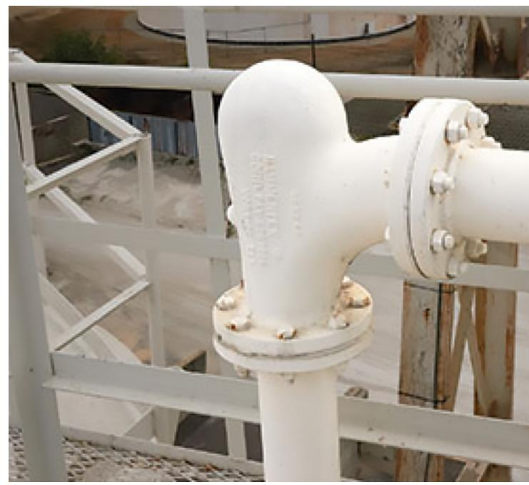
Action Supply, Sharon Hill, PA, eliminated surprise blowouts and associated repair costs after switching to short radius deflection elbows that minimize elbow wear.
