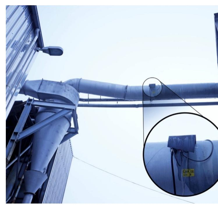
Highly sensitive GreCon spark detectors, type FM 1/8, are mounted on the exhaust duct and detect sparks and glowing particles.
