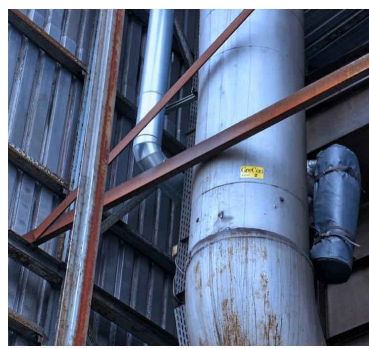
An automatic extinguishing device is mounted directly before the filter and eliminates risks of fire before they can cause damage.
