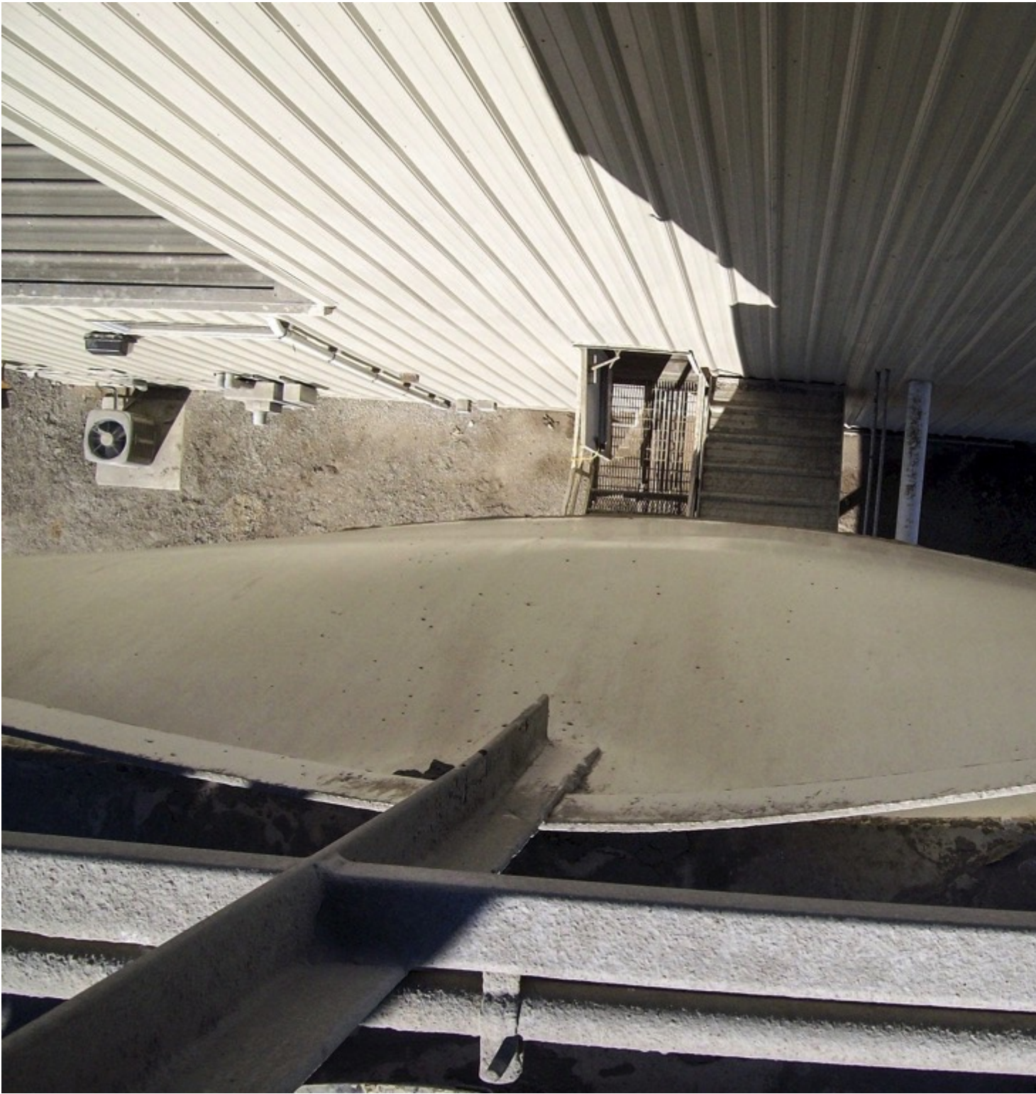
Silo walls bulged, due to increased internal pressures. (Pictures: ©Martin Engineering)
