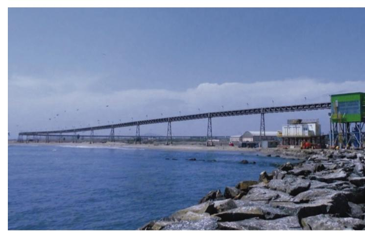
The pipe conveyor ends at the transfer tower, where the material is transferred to the ship loading system.
