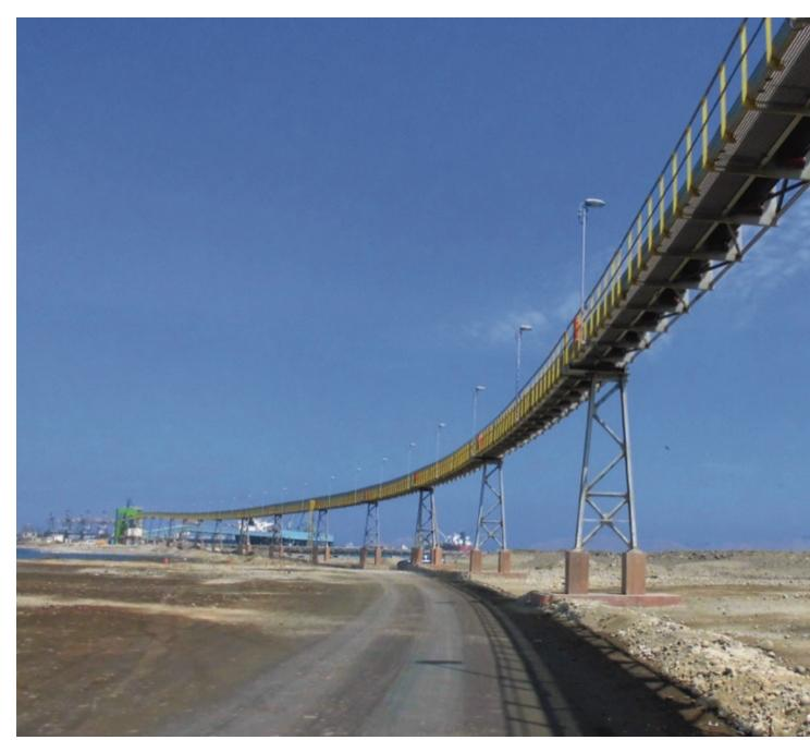
Beumer Group supplied and installed a pipe conveyor with a centre distance of 3195 m. (Pictures: ©Beumer Group GmbH & Co. KG)
