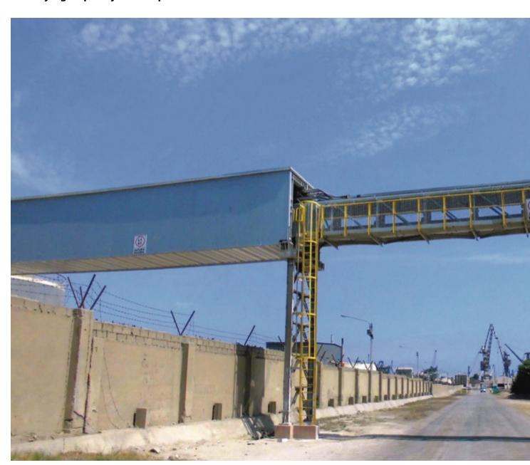
Just a short distance downstream from the loading point the pipe conveyor crosses the refinery area, where it had to be equipped with a fire-proof housing.
