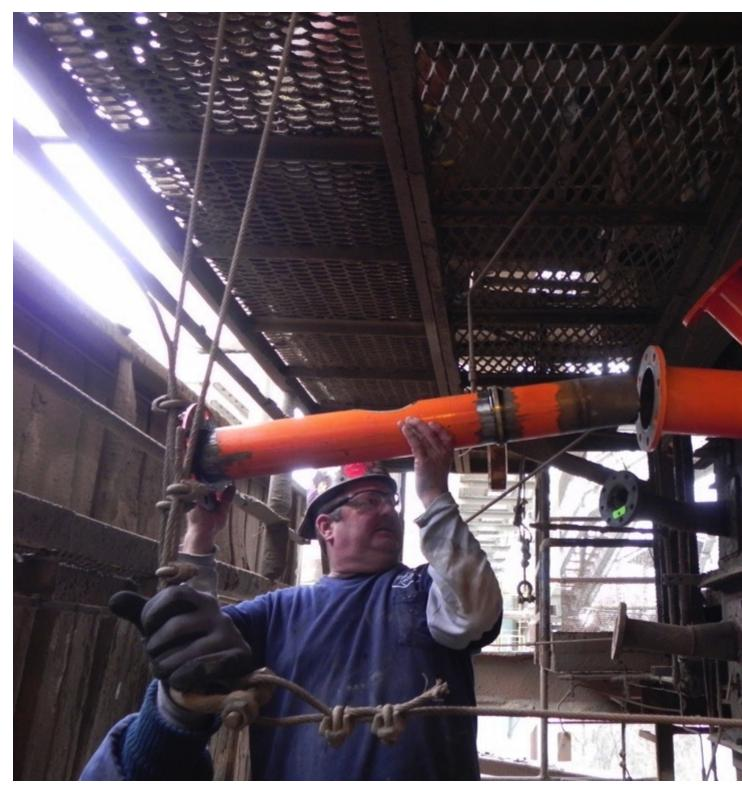
Avoiding confined space entry has eliminated much of the potential risk and shutdown time during nozzle changeouts.
