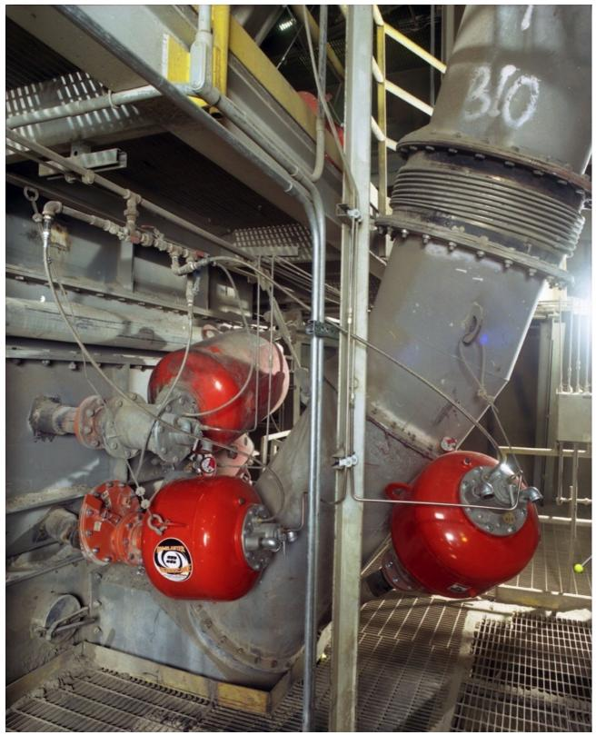
New air cannon valves produce about twice the blast force output of older designs, using approximately half the air volume.
