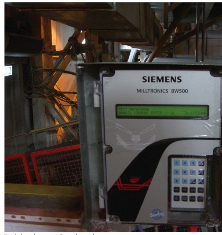
The belt scale relays information to the Milltronics BW500 integrator, which provides operators with belt speed, material flow rates, and other crucial information.
