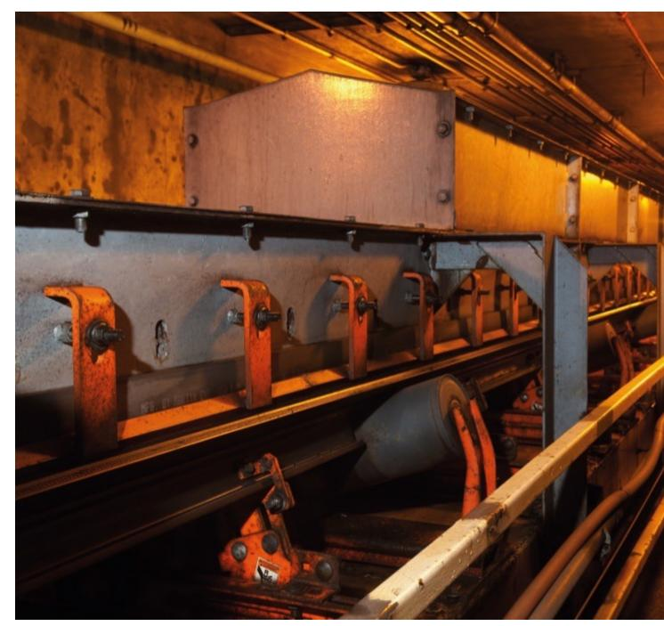
The new support system under the skirt board better supports the edges of the belt and helps eliminate sagging.
