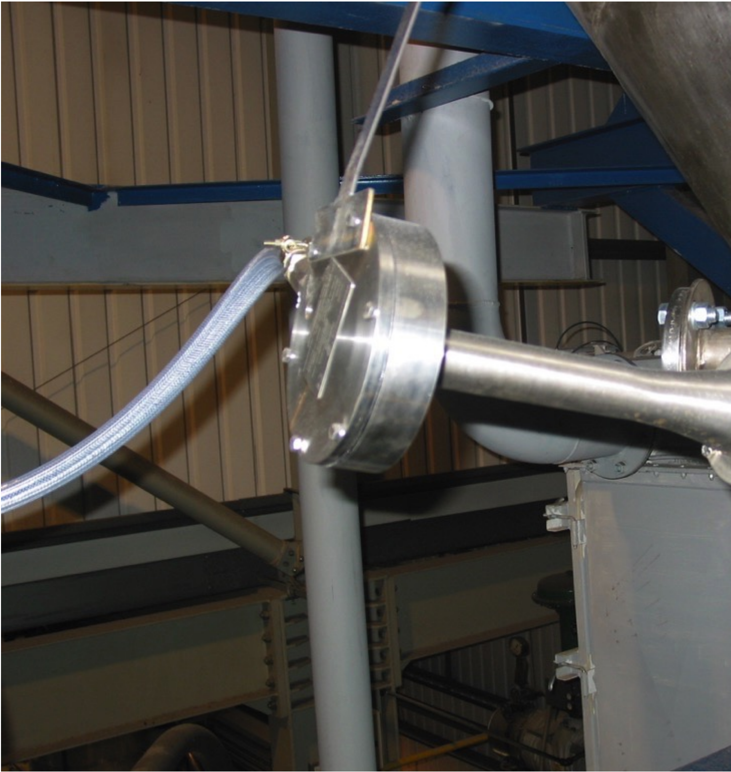
Typical installation of an acoustic cleaner at a hopper.
