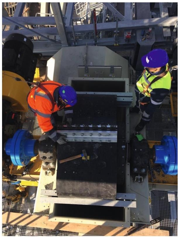
The technicians of BEUMER mount the steel cord belt with the BEUMER belt clamping connection.
