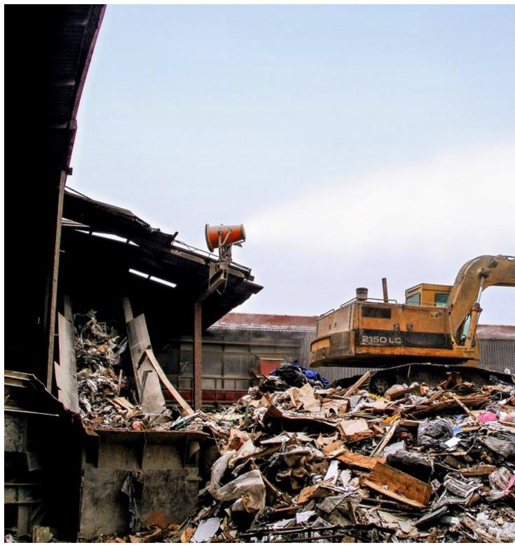
Landfills and recycling operations can achieve dust & odor control to save time and reduce potential additive waste.
