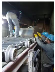
The specific design of the BEUMER system's cell strand facilitates the clean transportation of the clinker – no clinker can run out.
