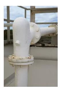
The Smart Elbow® deflection elbow installed in ready-mix plants prevents abrasive materials from impacting the elbow wall, eliminating worn elbows, related downtime and recurring maintenance costs.
