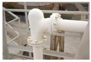
Action Supply, Sharon Hill, PA, eliminated surprise blowouts and associated repair costs after switching to short radius deflection elbows that minimize elbow wear.
