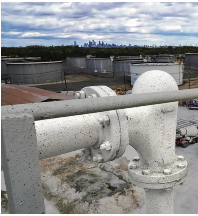
HammerTek short radius deflection elbows eliminated the need to weld or replace fail
