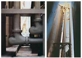
These 95' pipes were assembled on the ground and then stepped into their racks, greatly reducing costly crane time.
