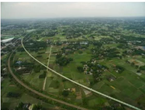
Project Sichuan: BEUMER Group built a 27 kilometre long conveyor system through hilly terrain and unstable ground.
