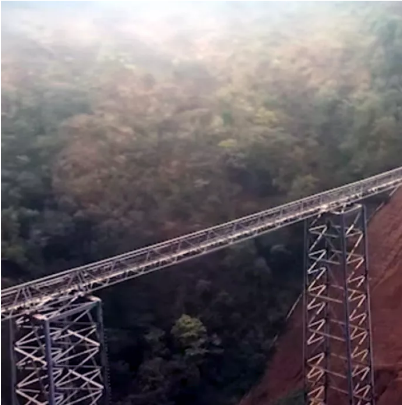
Fig. 8: Conveyor crossing gorge at 50m elevation
