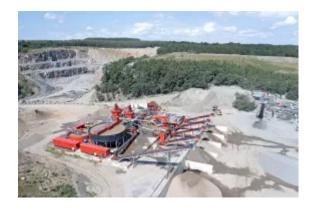
This new pioneering plant at Swerock's site in Blentarp processes feed material at a rate of 250tph to reduce the organics content in the output.
