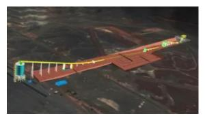
The F'Derick project in Mauritania. From right to left, the primary and secondary crushing stations, leading to the transfer tower and train loading station via a network of conveyor installations. This complex system is the result of our expertise in delivering complex bulk material handling systems. (Picture: ©TAKRAF GmbH)
