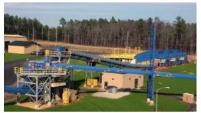
Bruks Siwertell's equipment deliveries include a drum chipper, screening and size reduction equipment, a radial stacker, as well as the complete conveyor system. (Picture: Bruks Siwertell Group)
