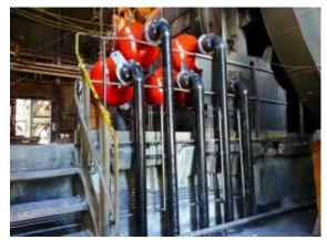
11.5 mm pipes lead down to holes drilled into the concrete floor, then continue under the subfloor.
