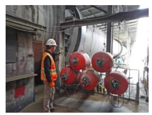
Valves face outward for convenient maintenance, requiring no tank removal to service them.
