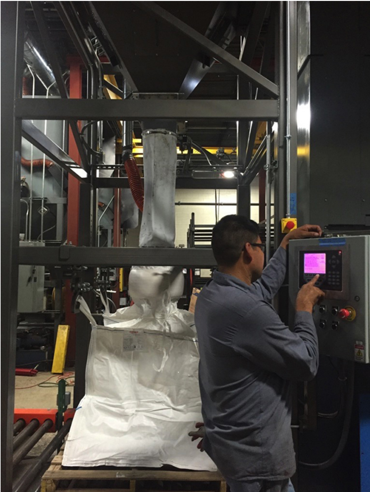
Fig. 2: Bulk Bag Filling and Finished Product, Includes Controls.
