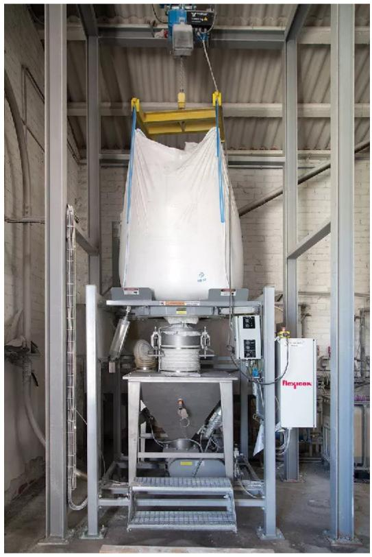
The powder flows dust-free into the hopper and into the following 38 m long pneumatic transfer line.
