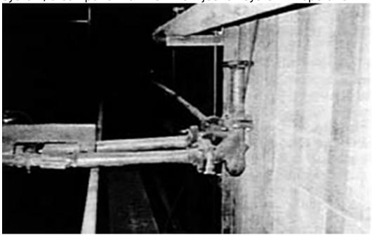
The solution to conveying system elbow wear at North Incinerator: Smart Elbow® deflection elbow in use in the lime injection conveying system.
