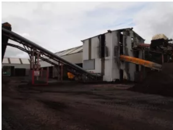
Dunlop BV XS conveyor on the left stopped the spread of fire.
