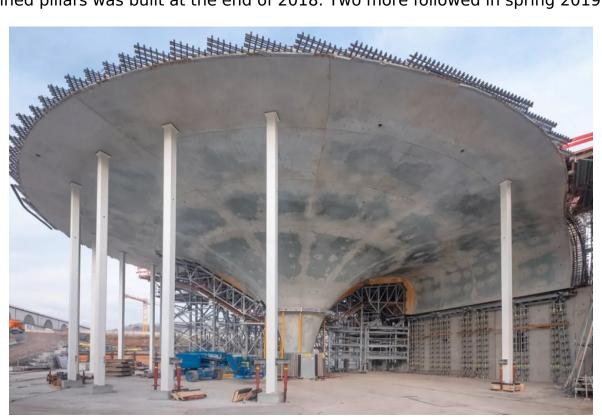
The sulfides in the granulated blast-furnace slag give the pillars a blue tint, which will disappear over time.
