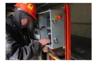
A technician wires the panel to control the Roll Gen system.
