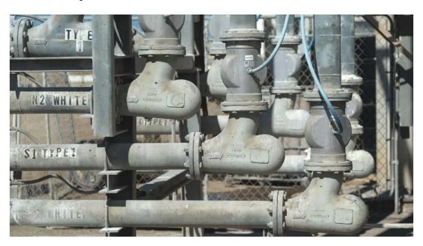
At this concrete production plant, the compact dimensions of the tightradius Smart Elbow design minimize space requirements compared to long-sweep elbows.
