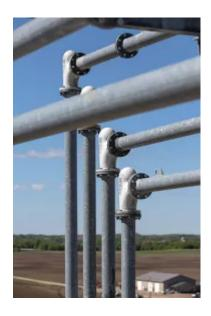
These Smart Elbow deflection elbows reduce aeration of dry cement powder moving through the pneumatic lines, decreasing dust collection demands.
