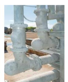
The tight-radius Smart Elbow deflection elbow provides a controlled flow, which is especially advantageous when conveying dusty materials such as cement or fly ash.
