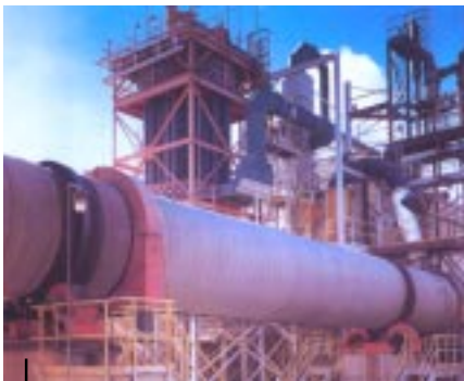
Rotary Dryer System
