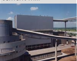
limestone storage and silos for additives
