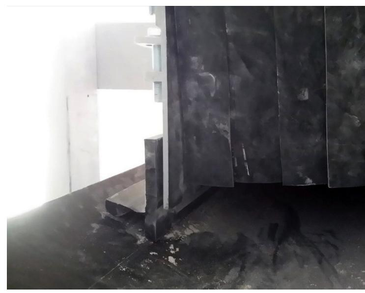
Dust curtains slow down the air flow and reduce fugitive particle emissions.
