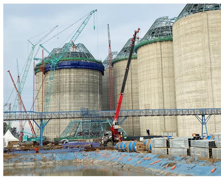
The solution for Komipo includes eight coal silos of each 55.000 m<sup>3</sup>, working together as one efficient fuel management facility and connected through networked conveyor systems party supplied by Rollent. (Picture: ©ESI Eurosilo B.V.)
