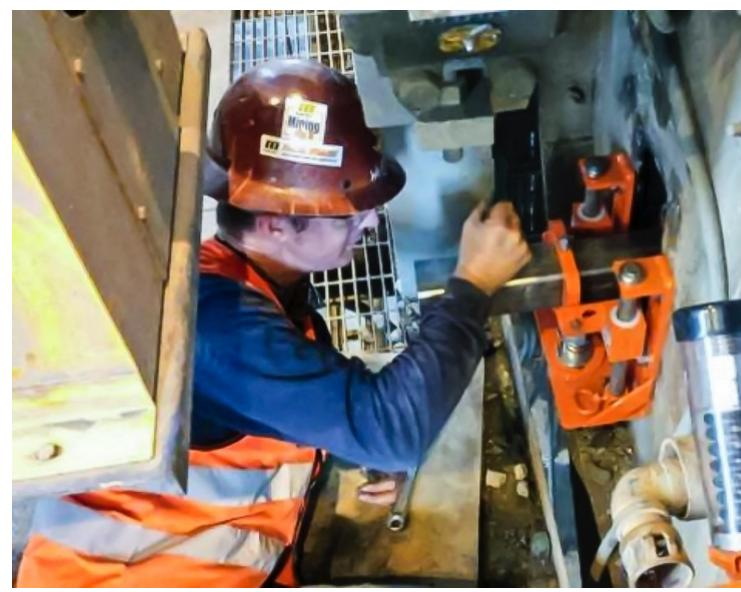
Martin Engineering replaced existing primary cleaners at sixteen discharge points, fitting them with low-adhesion urethane blades.
